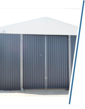
A tent hall has been constructed on the plot, with a load-bearing structure made of aluminum-steel (Al 234x100x3 mm). The roof is covered with a PVC tarpaulin, with a gable design and a roof pitch angle of 15°. The walls are covered with trapezoidal sheet metal T-35, 5 mm thick, arranged vertically. The hall has an area of 239.46 m², a width of 9.5 meters, and a length of 25.21 meters.
